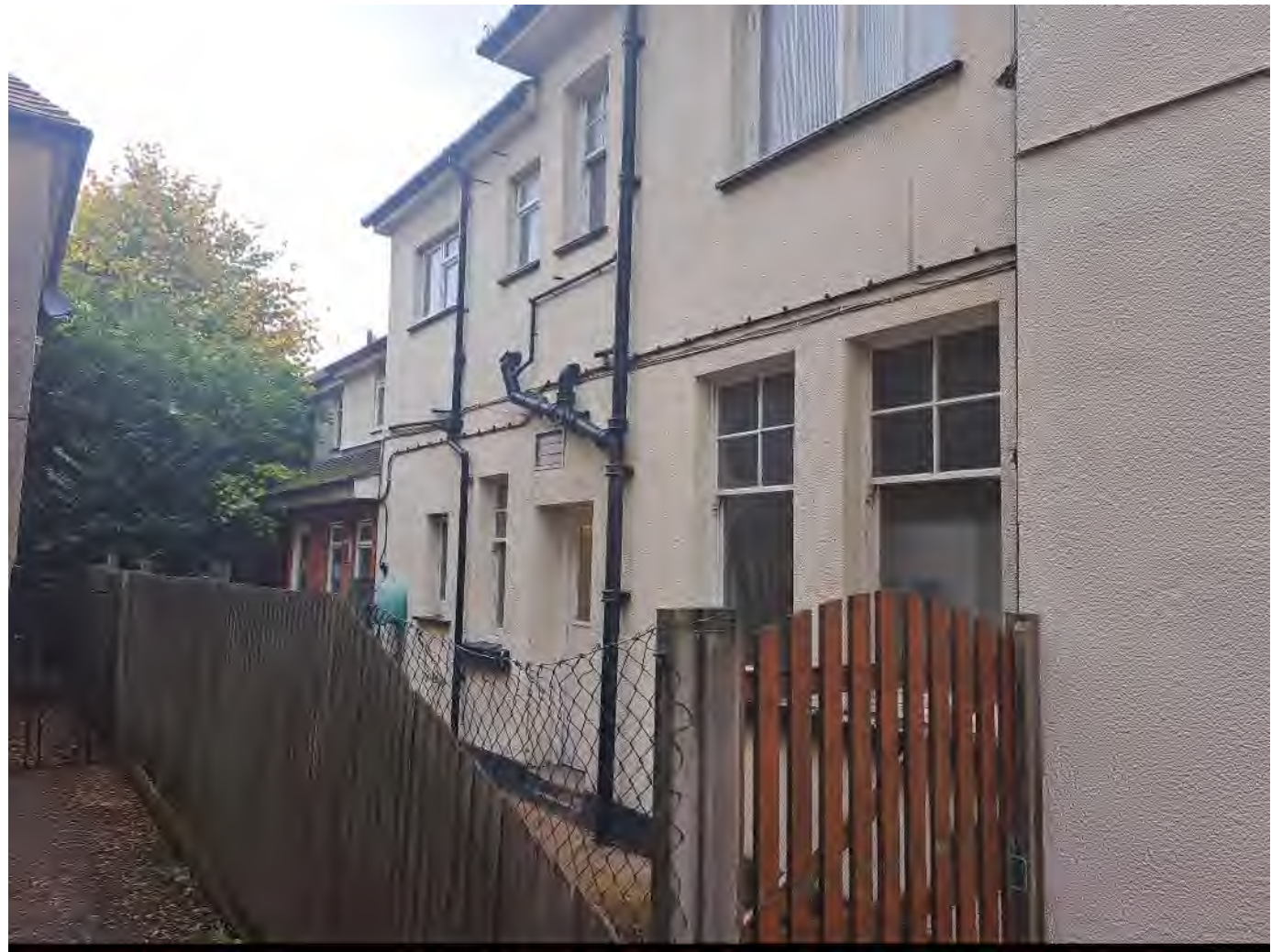
Flank elevation of 9 Imperial Avenue
